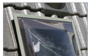
Tint (on tile roof profile)
